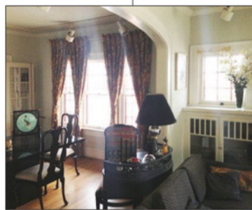
One of the most dramatic features of the existing house was the lone elliptical arched cased opening that occurred only between the living and dining room.
