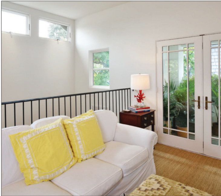
At the top of the stair hall / gallery, an intimate master sitting room leads to a private veranda. To lend a visual lightness throughout the second floor aerie, a kerfed drywall detail was used instead of wood casing for the doors and windows.
