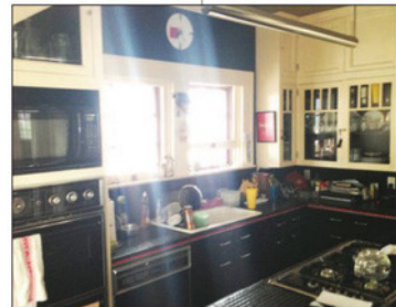
The existing kitchen renovated in the 1980s, neither narrow enough for a galley kitchen nor wide enough for a proper island, was expanded to accommodate a usable island flanked by custom full-height Shaker-style cabinets. The original single-hung sash windows above the sink fully retract into a pocket in the exterior wall.
